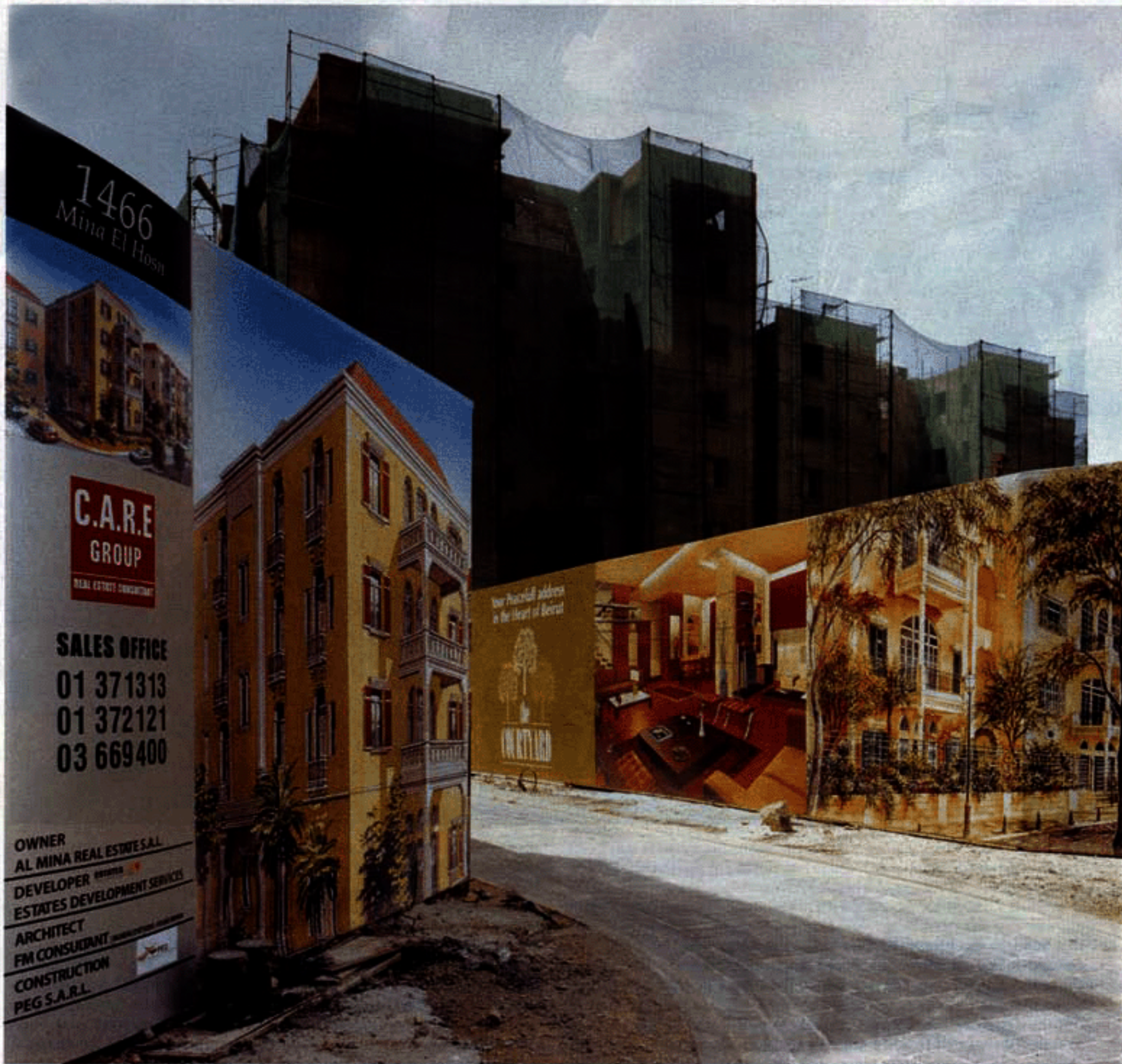
BEIRUT'S FUTURE Fences surrounding the construction sites for new residential buildings
