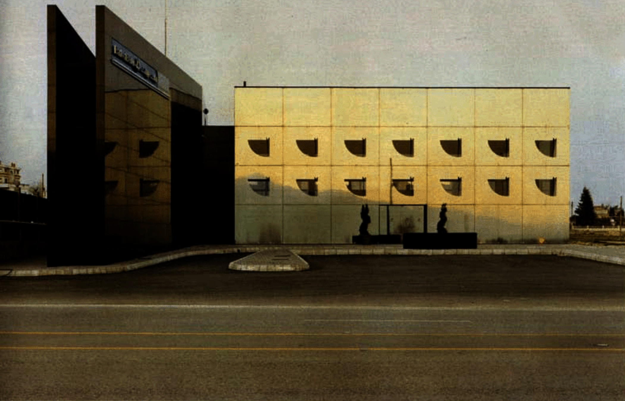
BANKS AND A BLACK BOX One of two banks designed by Khoury in Chtaura, a town close to Lebanon's border with Syria. Opposite: Black Box Alzone, a Khoury nightclub in Beirut. At the end of the steel arm, a screen projects live images from inside.
